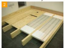
Begin by fixing the sheet ply on support battens ensuring that the ply is 30mm below the top of the joists. The trap requires the ply to be mounted flush with the joists. Make the raised ply the same length as the linear gulley.
