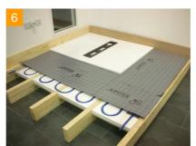
JUPITER system foil can be then unrolled over the remaining exposed heating system. This protects the heating system from the Screed Replacement Tile adhesive.
